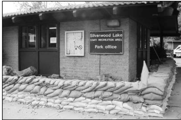
Figure 9. - Structure protection for building in Silverwood Lake 9
