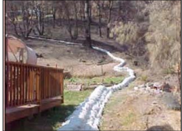
Figure 1. – Sandbag barriers placed to protect home in Jones Valley, CA 9
